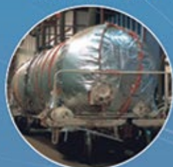
Tank Car Repair
